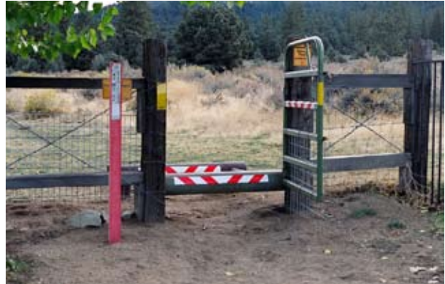
Figure B5. OHV barricade at equestrian gate. (There is no trail in this area.)
