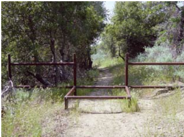
Figure 22. This nonmotorized trail barrier gate allows pedestrians and stock to pass through. The gate is flanked by a steel rail fence to prevent people from skirting the gate.
