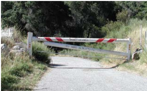
Figure 19. Standard Angeles National Forest road gate. Note that large rocks and berms have been placed to block entry around the gate.
