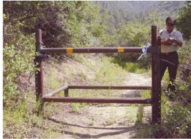
Figure 23. This nonmotorized trail barrier gate is shown with the upper bar closed, closing the trail to all traffic. A wire fence is attached to the gate to prevent people from skirting the gate.
