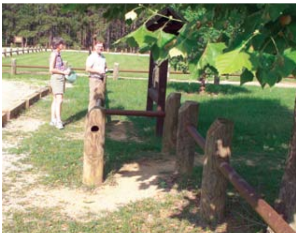
Figure 18. This gate has a single right angle turn and may not be as effective at keeping motorcycles out of an area.
