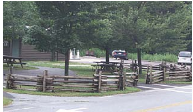
Figure 14. Double post stacked rail fence.
