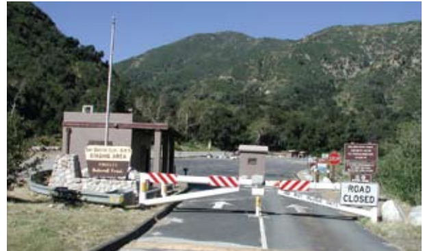
Figure 20. This double gate is used at an OHV area.
