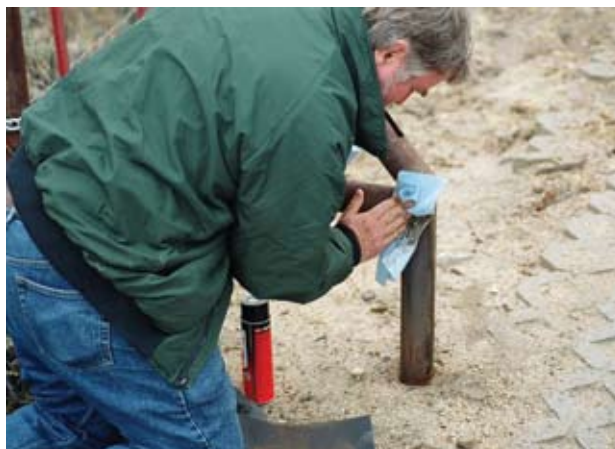
Figure B8. Clean residue off the surface using a quick drying degreaser/cleaner such as brake parts cleaner. Follow manufacturer's directions for use.
