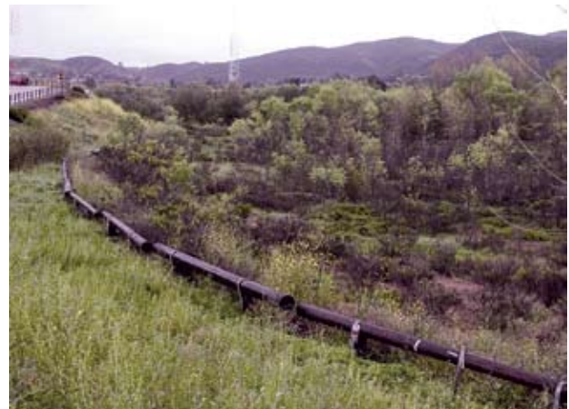
Figure 1. Telephone pole guardrail.
