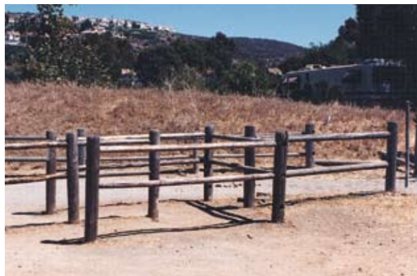
Figure 17. This wooden fence includes two right angle turns. The width of the opening is a maximum of 32 inches (nonaccessible).
