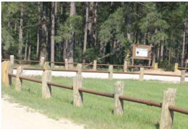
Figure 8. This wood post and steel pipe rail fence keeps motorcycles and ATVs on the road and off the grass. Note the trail entrance in the background.
