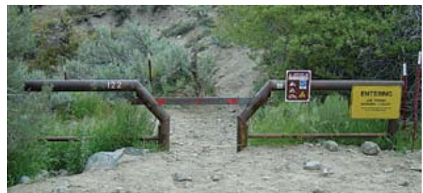
Figure 21. This width-limiter gate is used at trailheads to block certain vehicle types and to allow access by other types. A cross-bar is in place to close the trail to all uses.
