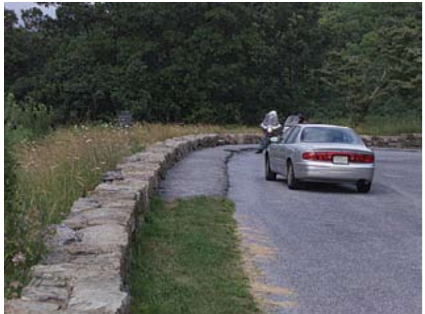
Figure 15. This low wall is held together with mortar; it is similar to using fieldstones to build a rock fence
