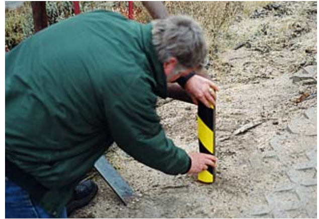
Figure B9. Measure and cut sheeting to correct size to assure proper fit.
