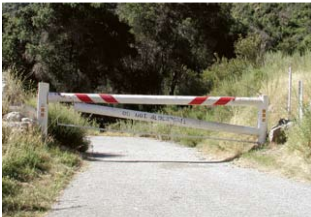
Figure B1. Striping points down toward the center of the road.
