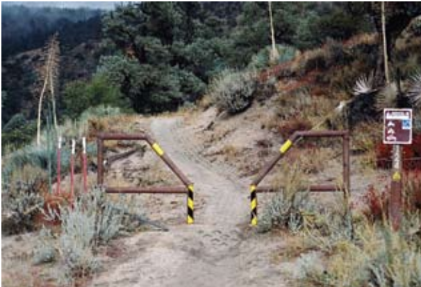
Figure 7. This width-limiter gate not only establishes the vehicle size that can be on the trail, it also marks the forest boundary.
