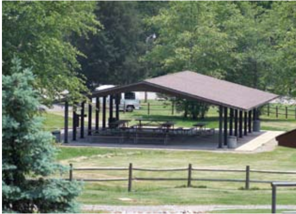
Figure 6. This wood post and rail fence surrounds a picnic area.
