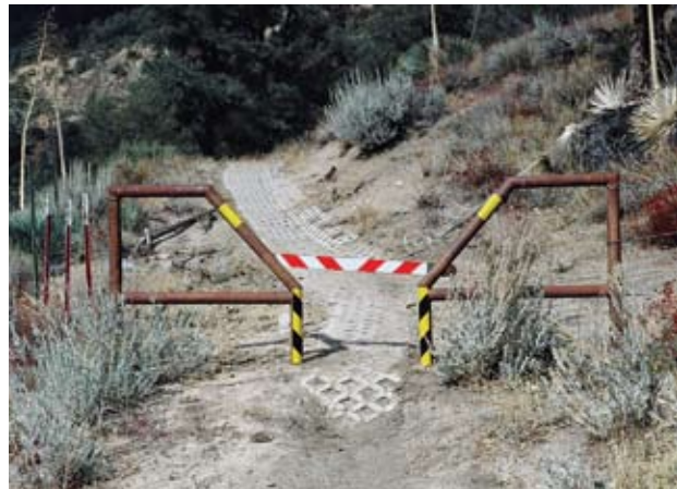
Figure A1. This width-limiter gate is closed to all traffic. The sides of the gate are attached to a wire fence.
