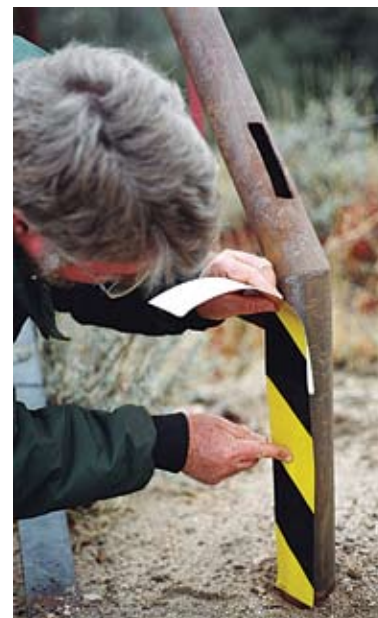
Figure B10. Note, remove backing slowly while pressing sheeting into place to avoid wrinkles.
