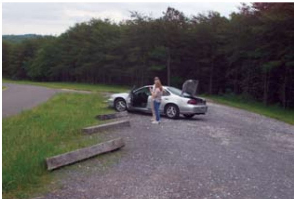
Figure 3. These 4- by 4-inch timbers are wheel stops that indicate parking spaces.
