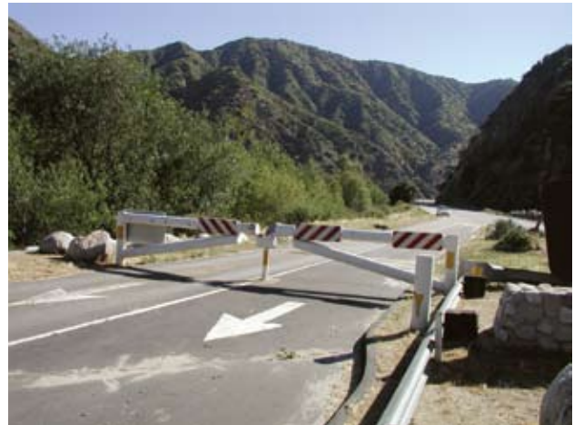
Figure B2. Shows striping on the back side of a double gate.
