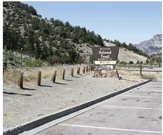
Figure 9. Bollards define the site's edge and separate the road and the parking lot.
