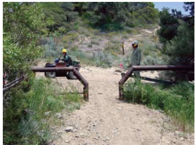
Figure 2. Steel framed width-limiter gate. This gate allows certain width vehicles through.
